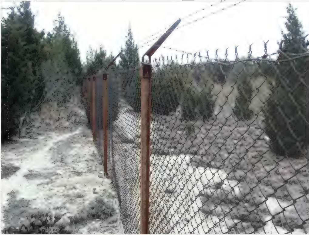
Figure 3.69. Outer fence, NIKE launch site. The launch site features a perimeter fence along its outside boundary and then adds an inner fence that encloses the missile magazines. This section of fence is in fair condition (Olmsted Center, April 2008).
